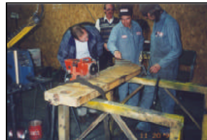
Wears out before cracking.
